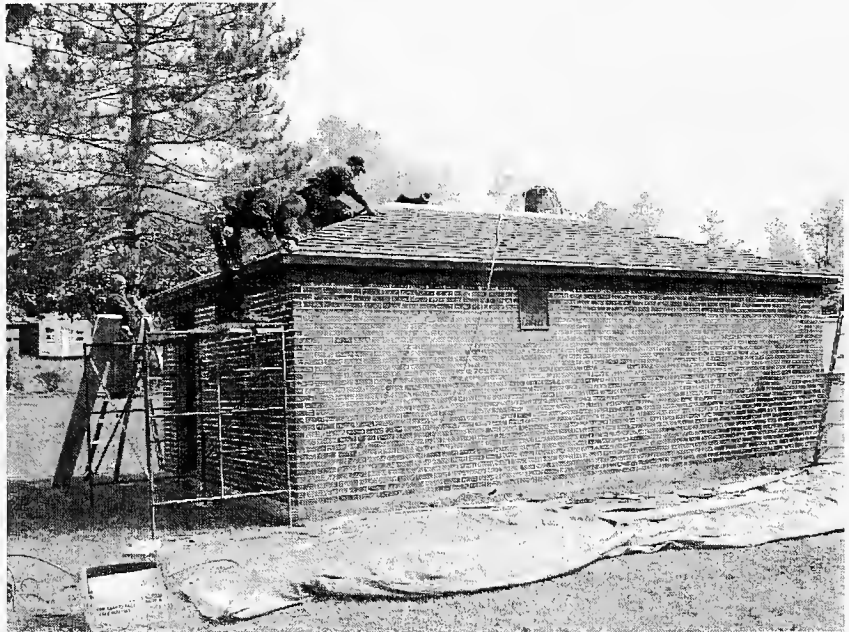
New Roof Installation at Jimtown CL2 Station
